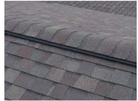
Ridge vent covered by shingles allowed
