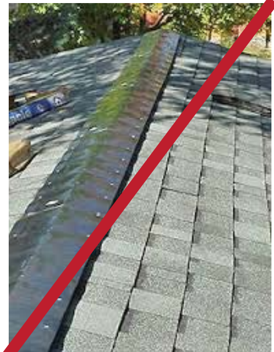
Ridge vent not covered is not allowed
