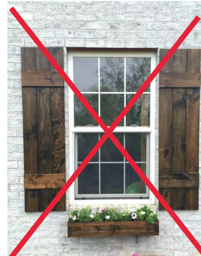
Incorrect mounting, lack of "operability"
